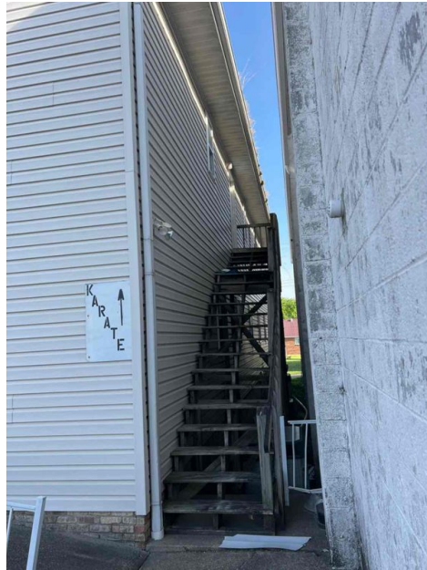
Right Side of Building
