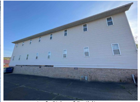
Left Side of Building
