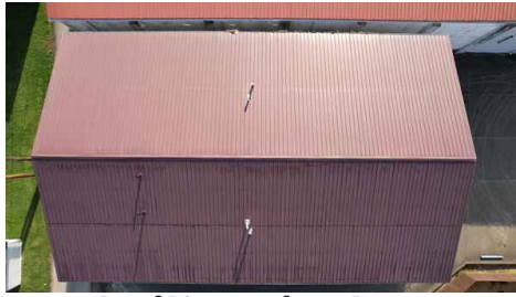
Roof Pictures from Drone
