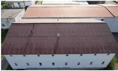
Roof Pictures from Drone
