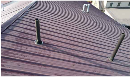
Roof Pictures from Drone
