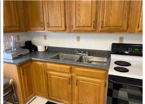
2nd Floor Kitchen Area - GFCI Protection Missing
