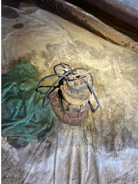
Old Sump Pump Present
