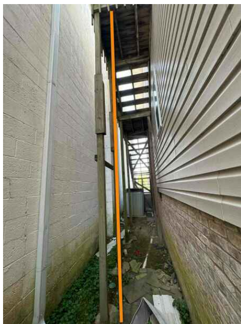
Side Steps 20 Feet Tall, Height Exceeds 4x4 Post Height Recommendations
