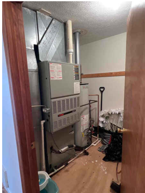
2nd Floor, Front Hallway - Right Unit
