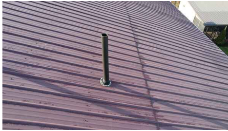
Roof Pictures from Drone
