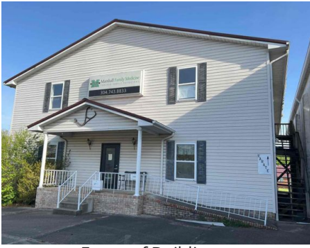
Front of Building
