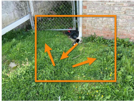
Rear Downspout Drains Near Building
