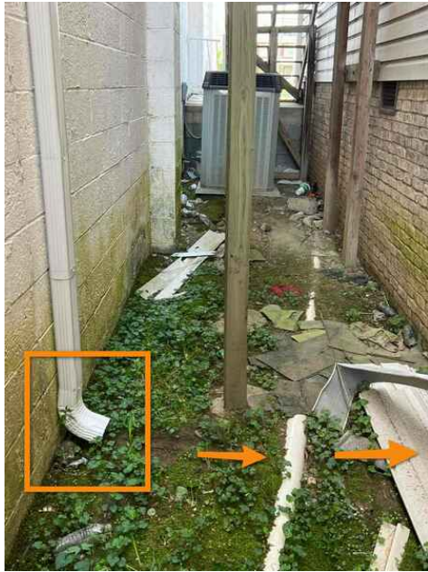
Downspout Drains on Ground Between Buildings
