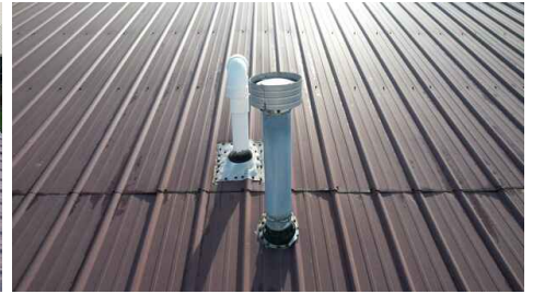
Roof Pictures from Drone
