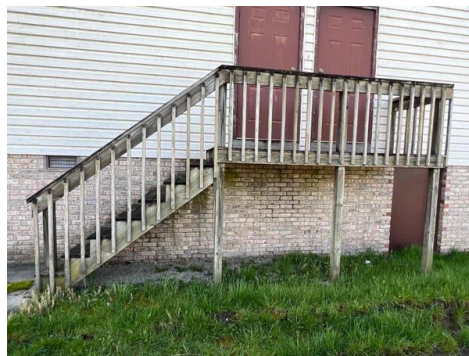
Rear Exterior Steps
