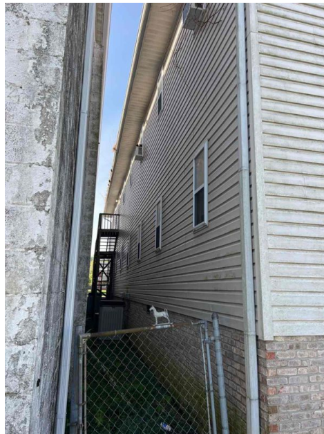
Right Side of Building
