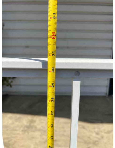
Front Porch Railing Height, Recommend 42"
