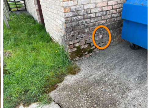
Left Side of Building, Sump Pump Discharge Pipe
