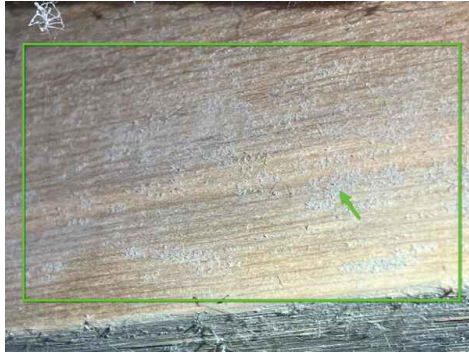
Crawlspace, Mold
