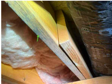
Crawlspace, Mold
