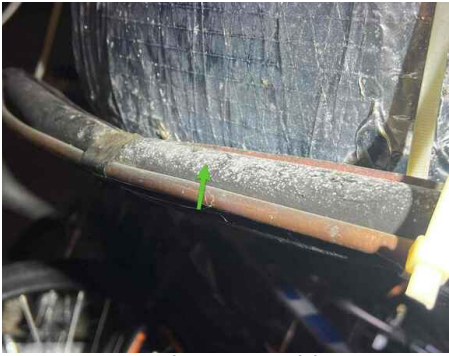
Crawlspace, Mold
