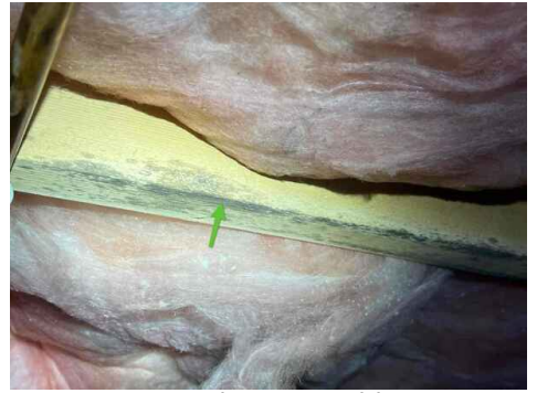
Crawlspace, Mold
