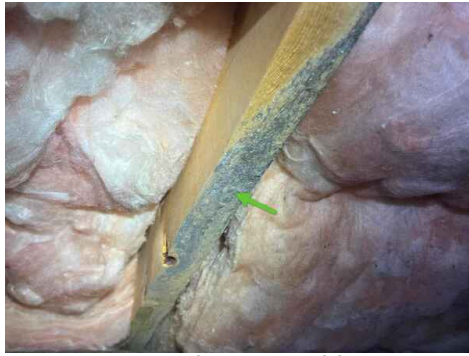
Crawlspace, Mold
