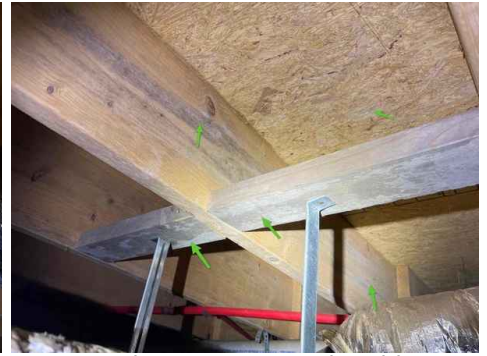
Crawlspace - Potential Mold - Example
