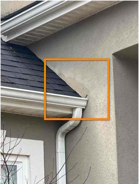
Front of House, Left Above Porch, Kick Out Flashing Missing
