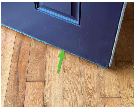
Front Door, Weatherstripping Damage
