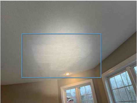
Master Bedroom, Evidence of Ceiling Repairs, Dry
