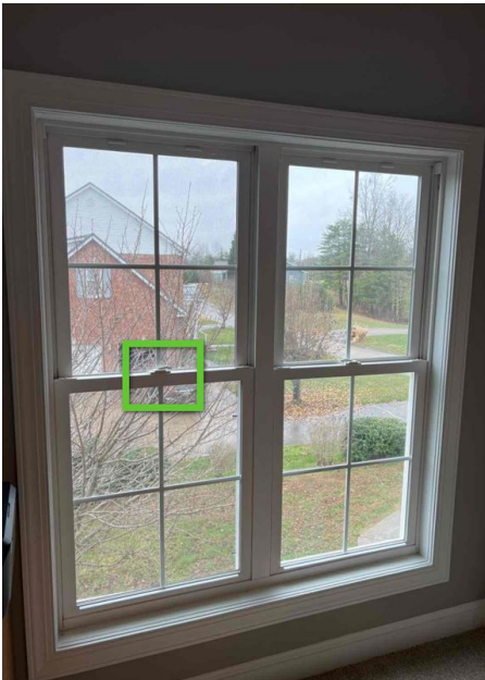
2nd Floor Family Room, Window Does Not Lock
