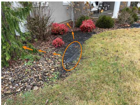
Front of House, Negative Grading - Example
