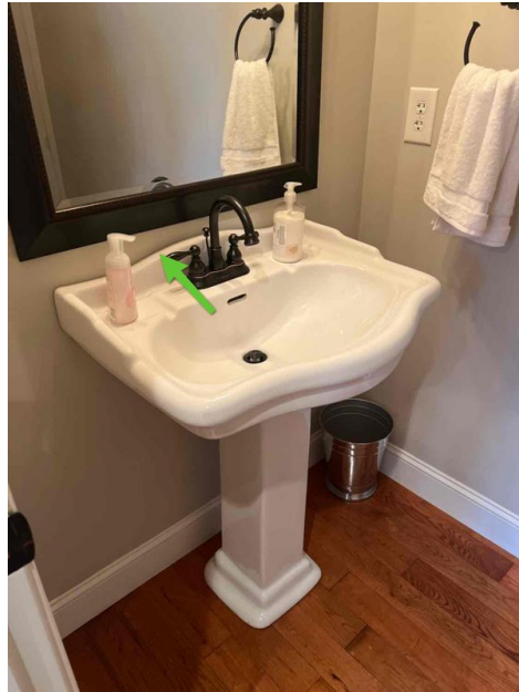
1st Floor 1/2 Bathroom, Sink Not Secure
