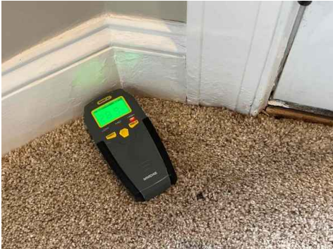
Master Bedroom, Rear Door, Wet & Deteriorated Baseboards
