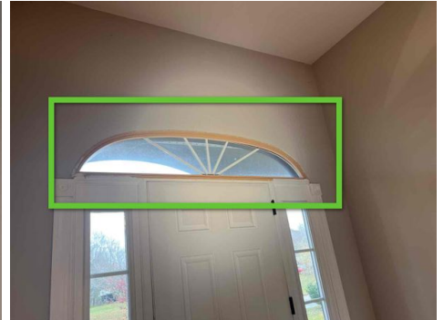
Front Door, Interior Trim Missing
