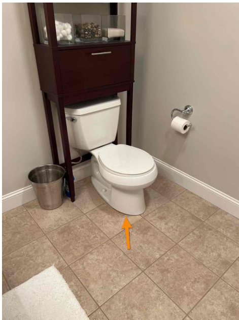
2nd Floor Bathroom, Toilet Not Secure
