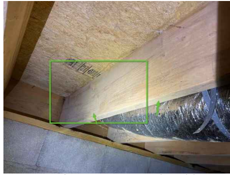
Crawlspace - Potential Mold - Example
