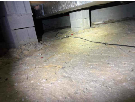
Crawlspace - Missing Vapor Barrier - Example
