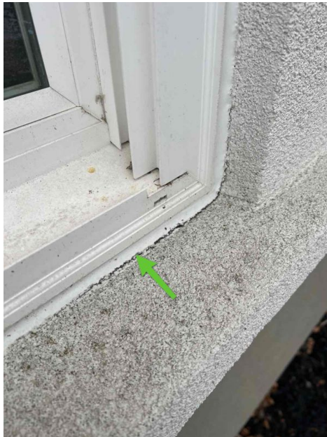
Recommend Sealing Exterior of Windows - Example
