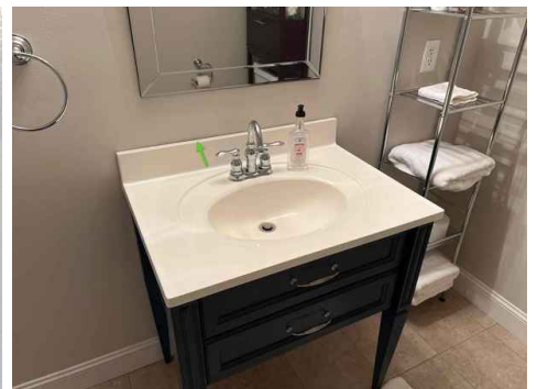
2nd Floor Bathroom, Vanity Not Secure
