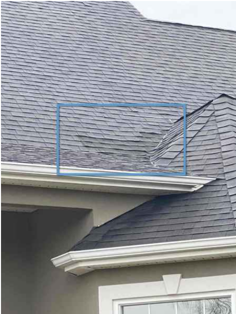
Rear of House, Evidence of Roof Repairs
