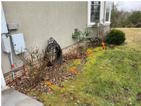
Right Side of House, Negative Grading - Example
