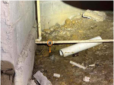
Crawlspace, HVAC Condensate Drains to Crawlspace
