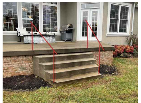
Rear Patio, Steps Missing Handrails
