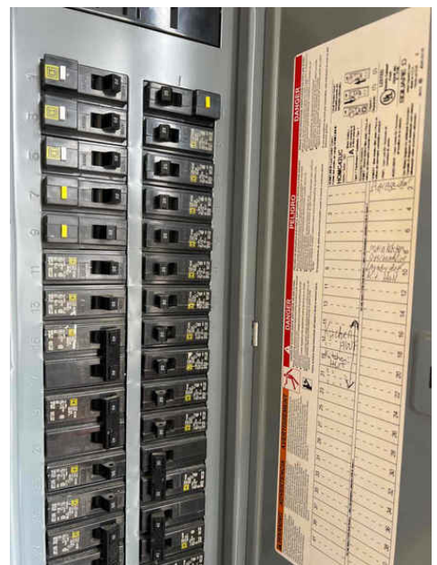
Attached Garage, Right Electrical Panel, Missing Full and Permanent Labeling
