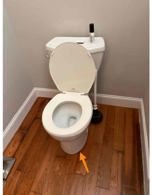
1st Floor 1/2 Bathroom, Toilet Not Secure
