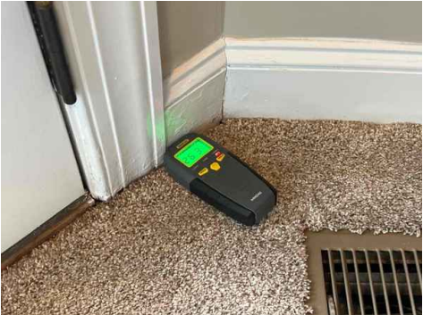
Master Bedroom, Rear Door, Wet & Deteriorated Baseboards
