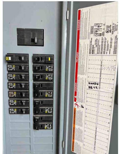
Attached Garage, Left Electrical Panel, Missing Full and Permanent Labeling
