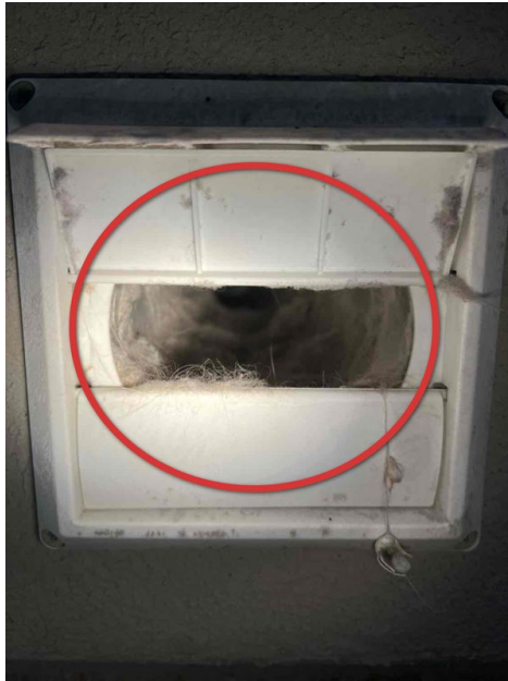
Dryer Vent Needs Cleaning
