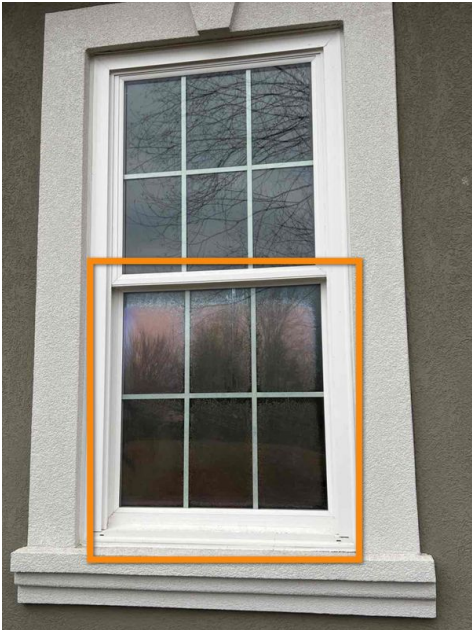
Attached Garage, Window, Failed Seal
