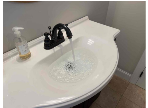
Jack & Jill Bathroom, Sink Not Draining Well
