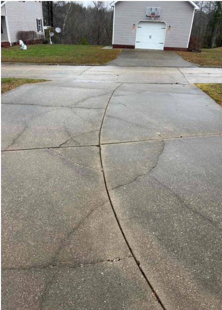
Driveway Cracks, Cosmetic, Recommend Sealing
