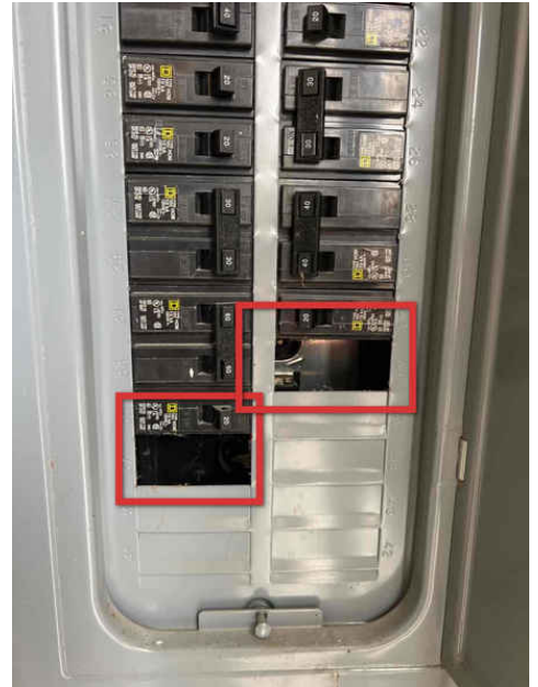
Attached Garage, Right Electrical Panel, Missing Knockouts
