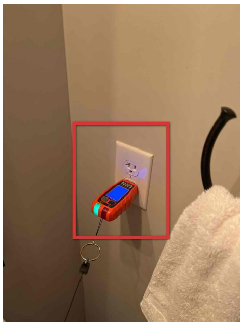
1st Floor 1/2 Bathroom, Receptacle Not GFCI Protected
