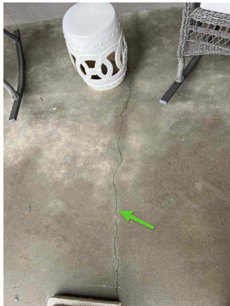
Front Porch, Cosmetic Cracks, Recommend Sealing
