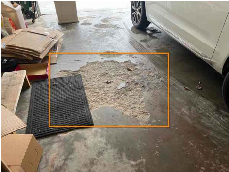
Attached Garage, Concrete Floor Deterioration - Example
