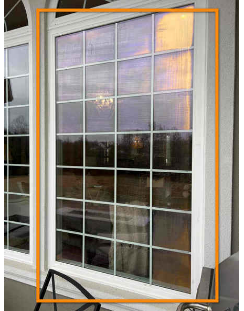
Living Room Rear Window, Failed Seal
