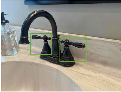
Master Bathroom - Right Sink - Handles Not Secure
