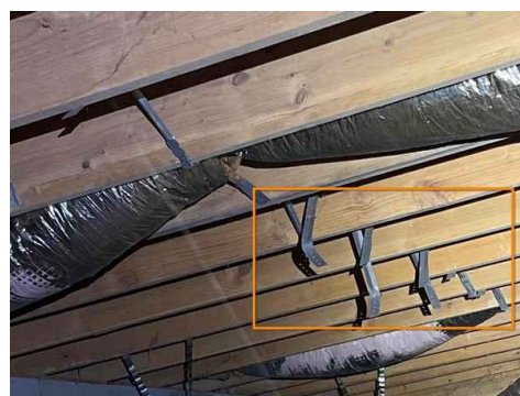
Crawlspace - Cross-bracing Not Installed - Small Example Only
