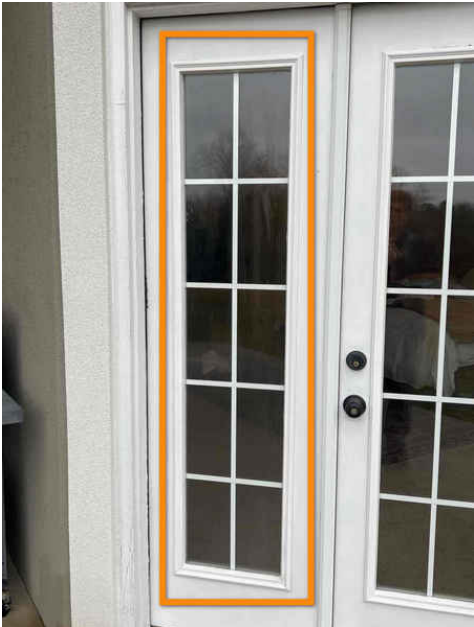
Master Bedroom, Door to Patio, Failed Window Seal
