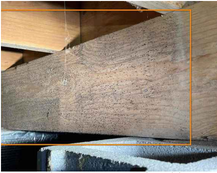
Crawlspace - Potential Mold - Example
