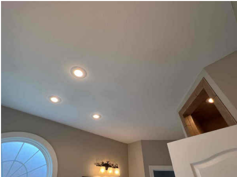
Master Bathroom, No Exhaust Fan Near Shower (In Toilet Room Only)
