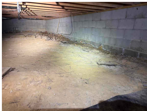
Crawlspace - Efflorescence, Water Intrusion - Example
