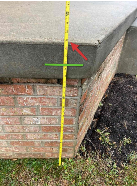
Rear Patio, Missing Safety Railings
