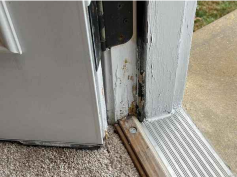
Master Bedroom, Rear Door, Severely Deteriorated
