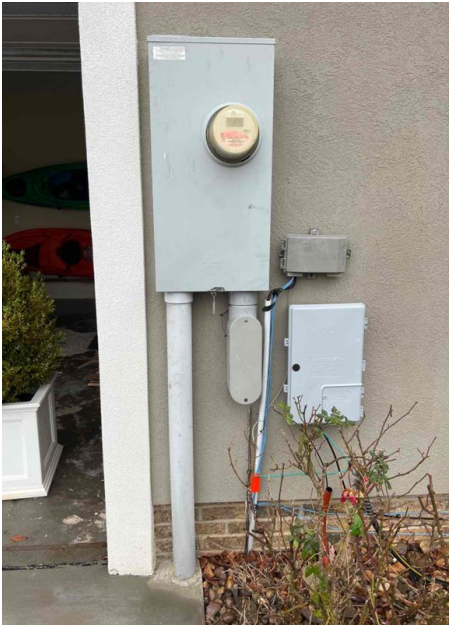
Power Service Entrance Cables, Right Side of House
