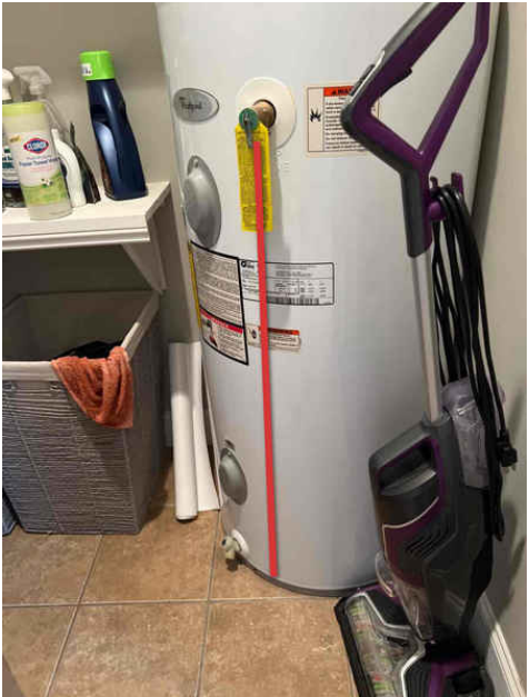
Master Bathroom Closet, Hot Water Tank, TPR Extension Missing
