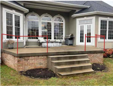
Rear Patio, Missing Safety Railings
