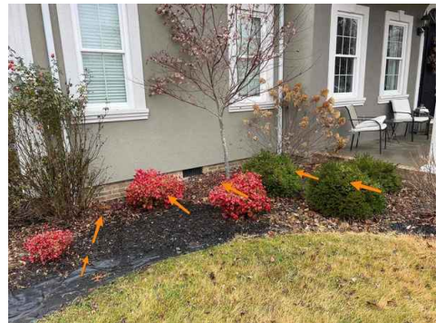
Front of House, Negative Grading - Example
