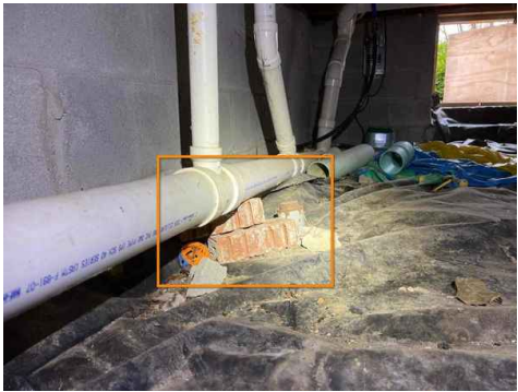
Crawlspace, Drain Line Improperly Supported
