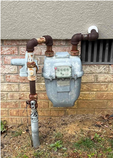
Main Fuel Shutoff, Left Side of House
