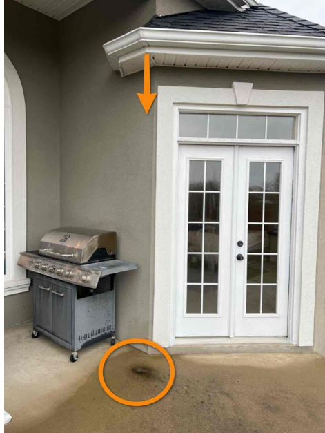
Rear Patio, Gutters Leaking
