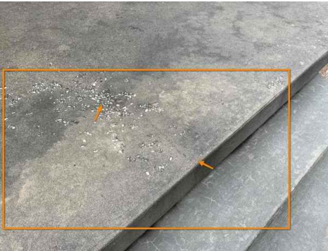
Rear Patio, Concrete Cracking
