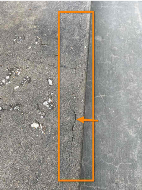
Rear Patio, Concrete Cracking
