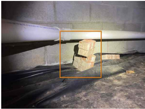
Crawlspace, Drain Line Improperly Supported
