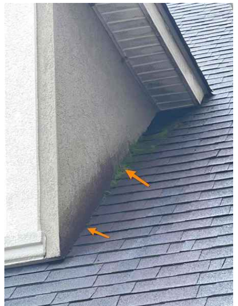
Front of House, Right Side of Smaller Dormer, Siding In Contact With Shingles
