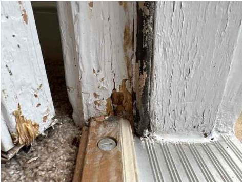
Master Bedroom, Rear Door, Severely Deteriorated
