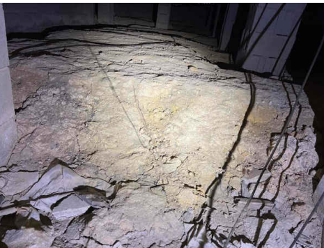
Crawlspace - Missing Vapor Barrier - Example
