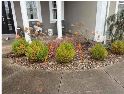
Front of House, Negative Grading - Example
