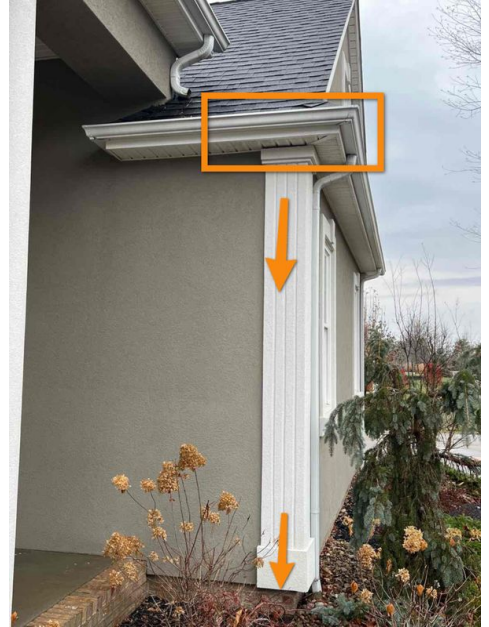
Front of House, Gutters Overflow
